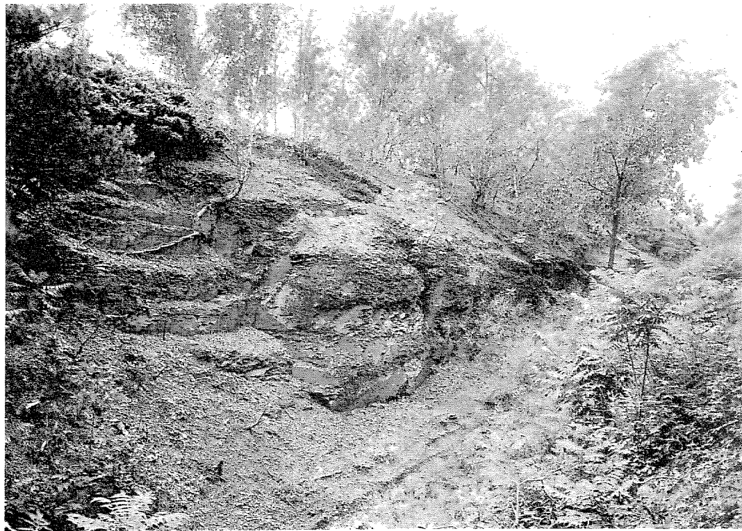
Figure 46 Cut in Esopus grit along (west side of) the John Boyd Thacher Park road. The jointing of the rock is well shown and also the ease with which it breaks up into a gravel. (Photograph by E. J. Stein)
